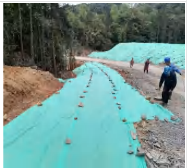
裸露地表临时苫盖
